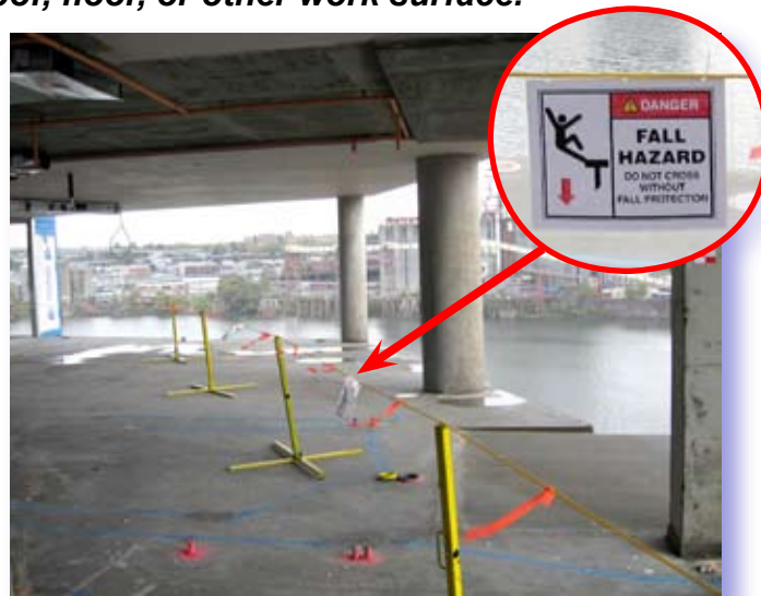
You can use a warning line to alert workers they are approaching an unprotected edge of a roof, floor, or other work surface. The warning line must be set up so that it eliminates the risk that a worker could fall over the edge. Signs and flagging emphasize the hazard.
